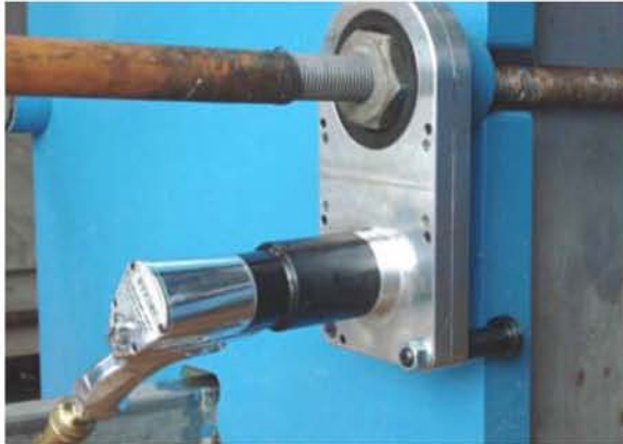
jGun-3 with ratchet link on heat exchanger
