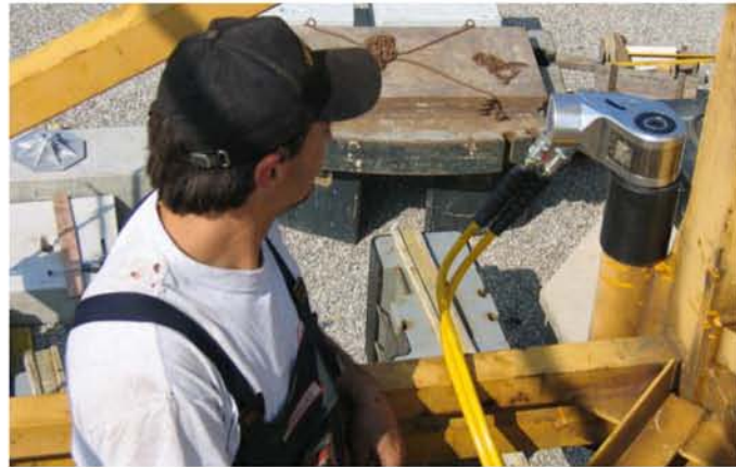
AVANTI-5 with DISC on a LIEBHERR 256HC at BKL
